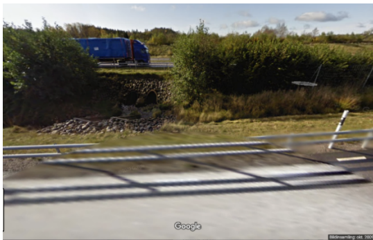
Figure 11. Culverts under E6 at Hogsbotorpsmotet. Retrieved from Google Maps. Image taken in October 2009, before the event.
