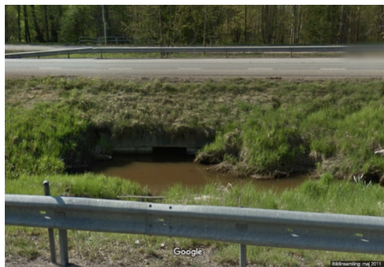
Figure 12. Stone culvert under E18 at IKEA, Värmland. Retrieved from Google Maps. Image taken in May 2011, before
