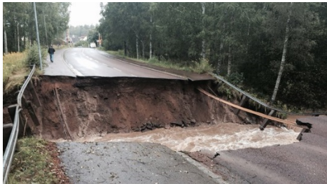
Figure 7. Lagmansgatan collapsed due to the heavy precipitation (Sveriges Radio, 2014-08-21)
