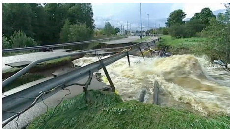
Figure 8. Östra Ringvägen was flooded (SVT nyheter Värmland, 2014-08-23)
