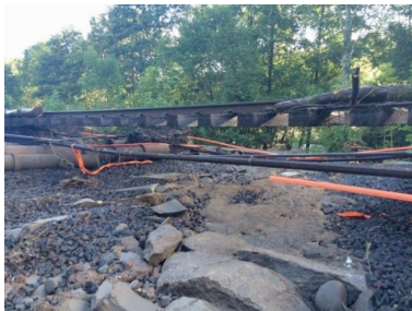
Figure 5. Railway embankment at Bohusbanan damaged (Småröd) (Bohuslänningen, 2014-08-21)
