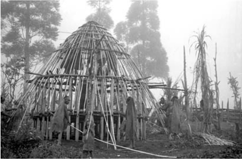
Figure 11. Cooperative work during construction of a Baruya couple's house (Wonenara, 1982).
